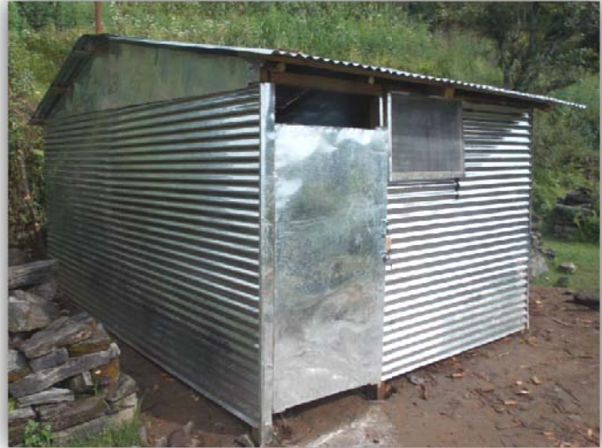
Fig. 2: Double slope temporary shelter at Panyali Village, Bageshwar district
