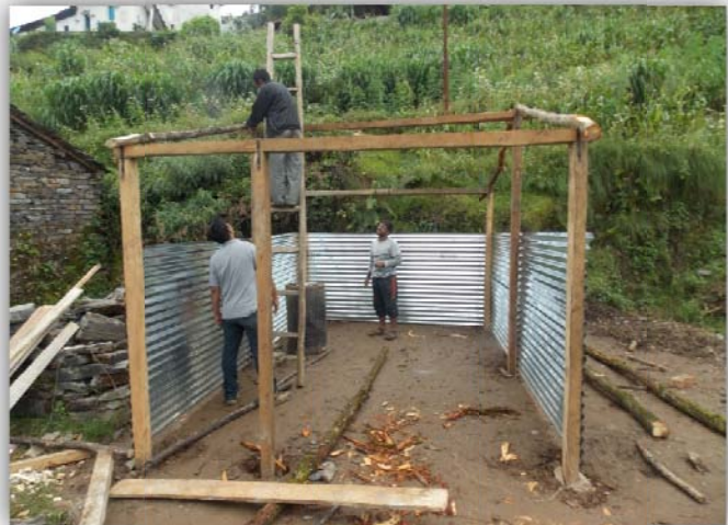
Fig. 3: Use of wooden section at the corners
